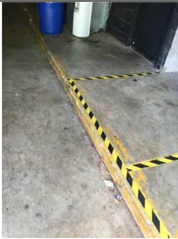
13. 1714 2 nd St: View of Lead-Based Paint on Yellow Concrete Curb in the Garage. XRF Reading No. 121.
