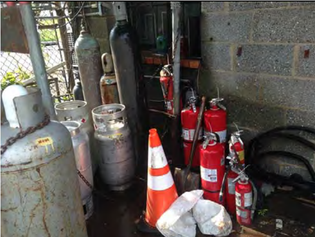
23. 1711 1 st St: View of Compressed Gas Containers and Fire Extinguishers.
