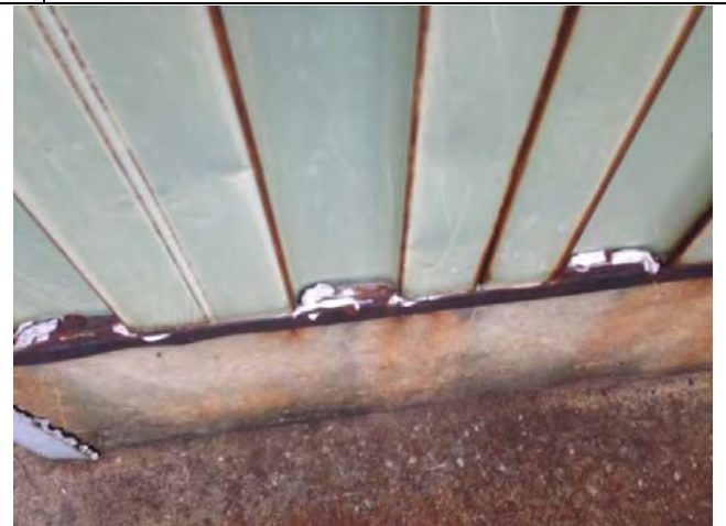
30. 2 nd and S St: View of Exterior White Siding Caulk (ACM). Sample No. AW-15.
