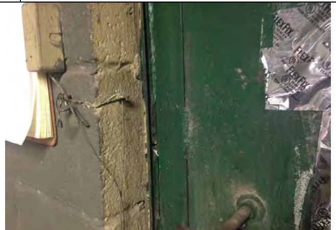
22. View of Lead-Based Paint on Green Metal Window Apron in the Rear Office. XRF Reading No. 9.
