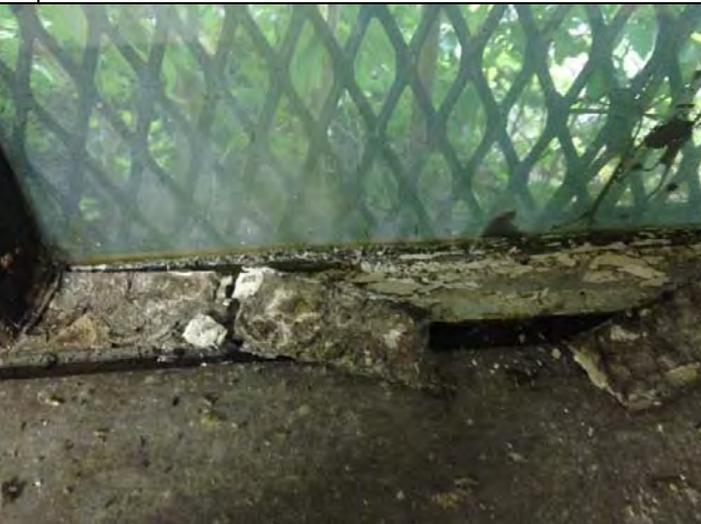
19. 2 nd and S St: View of White Interior Window Glaze (ACM) in the Warehouse Office. Sample No. AW-07.
