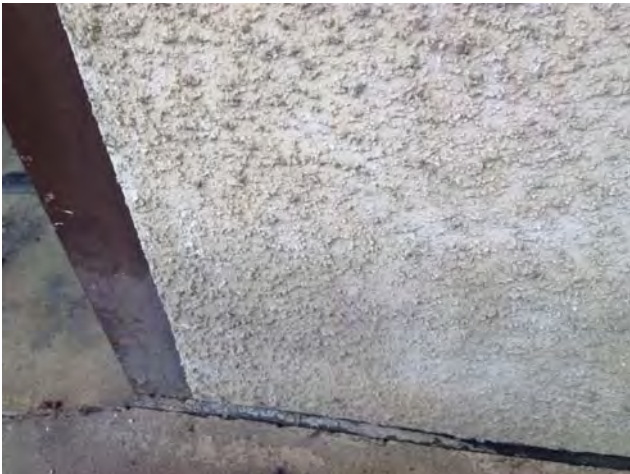
5. 1714 2 nd St: View of Exterior Wall Texture Coating (ACM). Sample Nos. BS-39 – BS-45.
